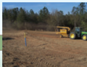
Reseeding the right-of-way
